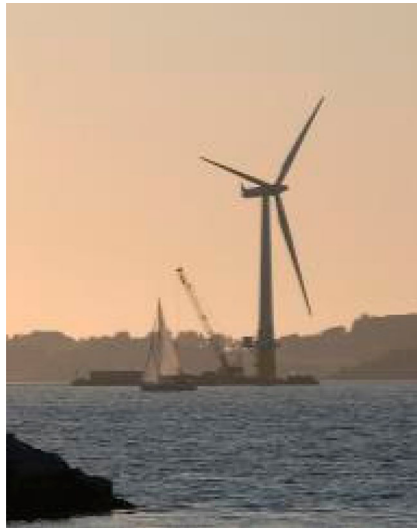
Figure 6. A floating 3 MW wind turbine. The ZCB reports envisage up to 100 GW of capacity in such machines in the deeper parts of UK territorial waters. Is this still AT? Credit: Statoil.
